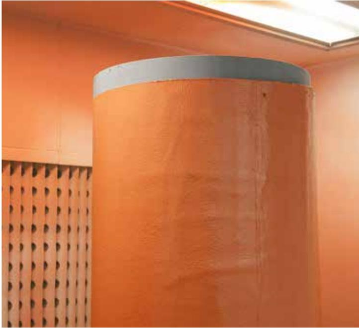
Belzona 5871 is a novel, two-component, polymeric, solvent free system providing a thermal insulation barrier with corrosion protection and thermal and sub-zero “cool-to-touch” properties.
