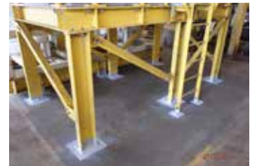
Sealed deck-support bolts
